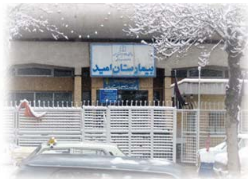
Figure 15. Omid Hospital in Mashhad, Khorasan Province. 76
